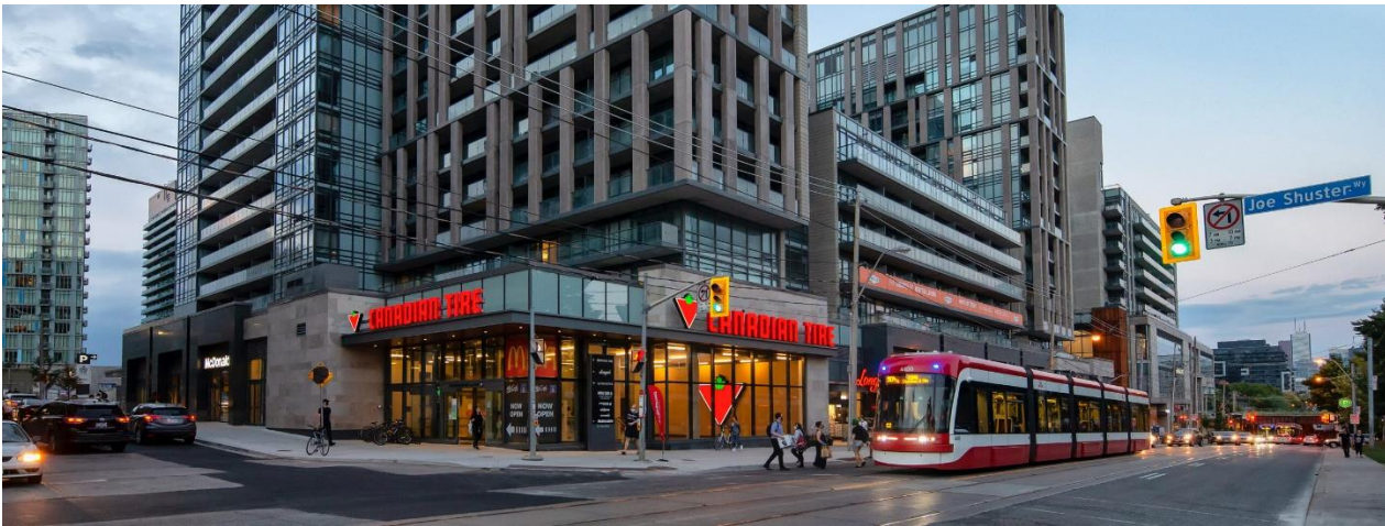
Figure 5-4: 1100 King Street West
